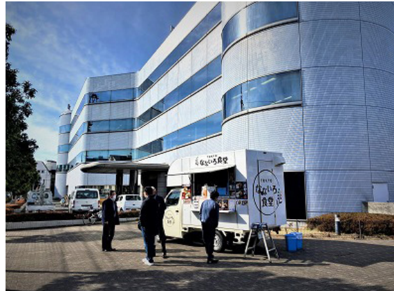
IIF Shinagawa Data Center
